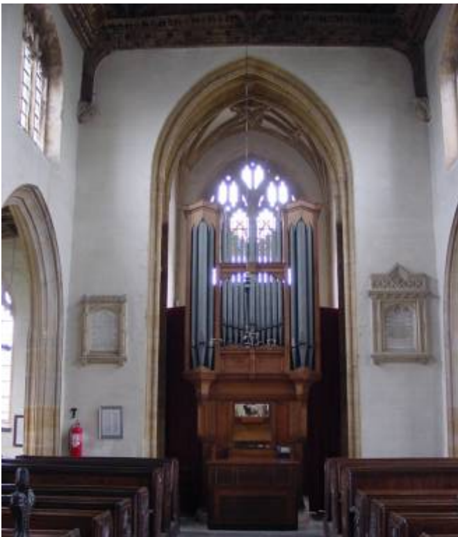
West end showing organ and full height of tower arch.
