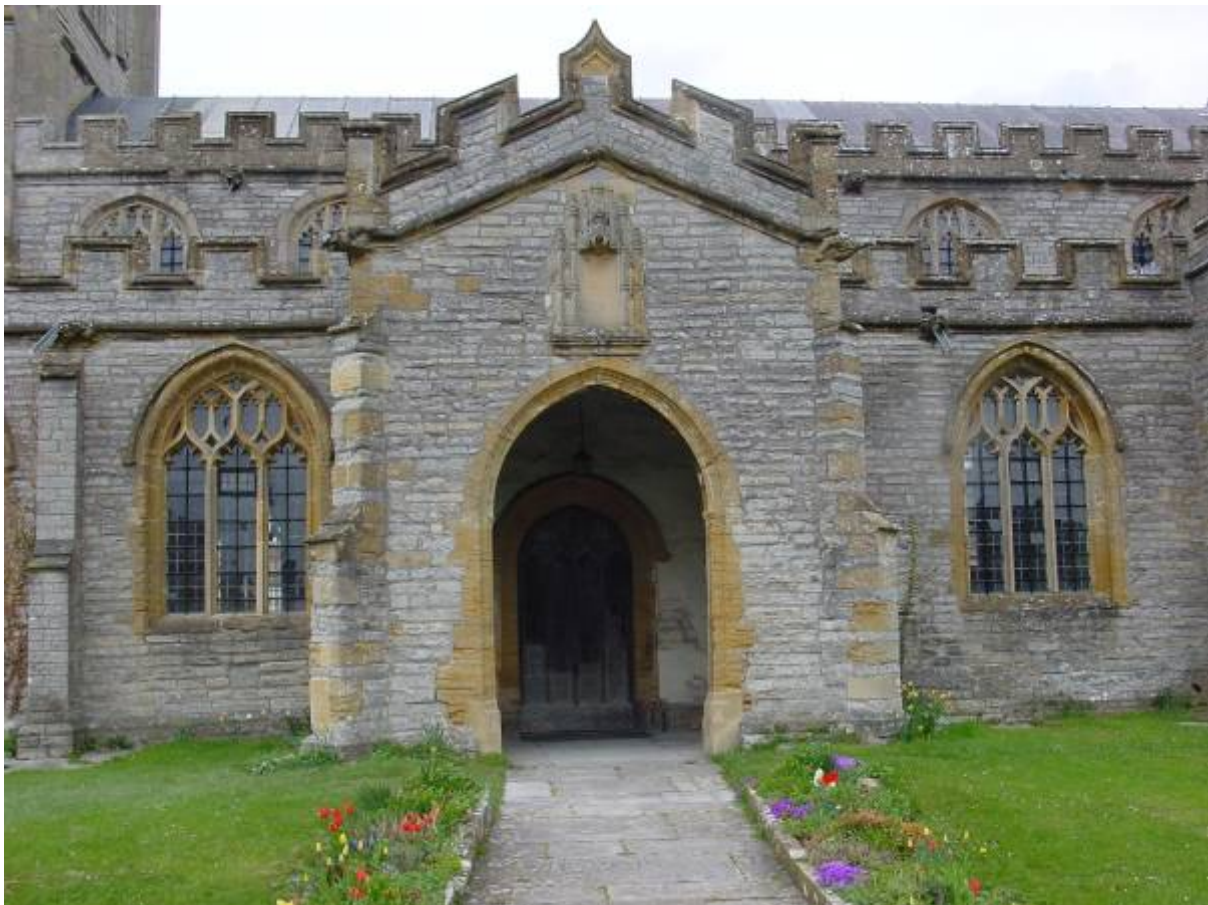
South Porch used as the main entrance.
